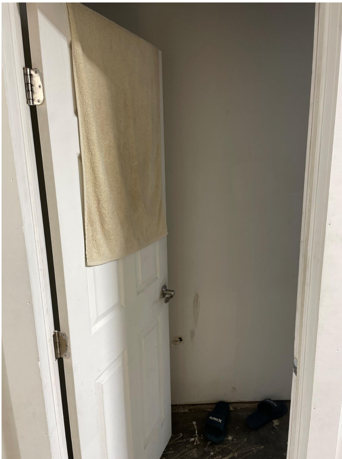
Hallway door to 1 st bedroom on the right.
