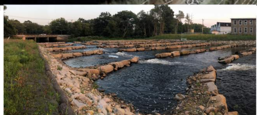
Boulder Weir Pool Example (Bradford Fishway)
