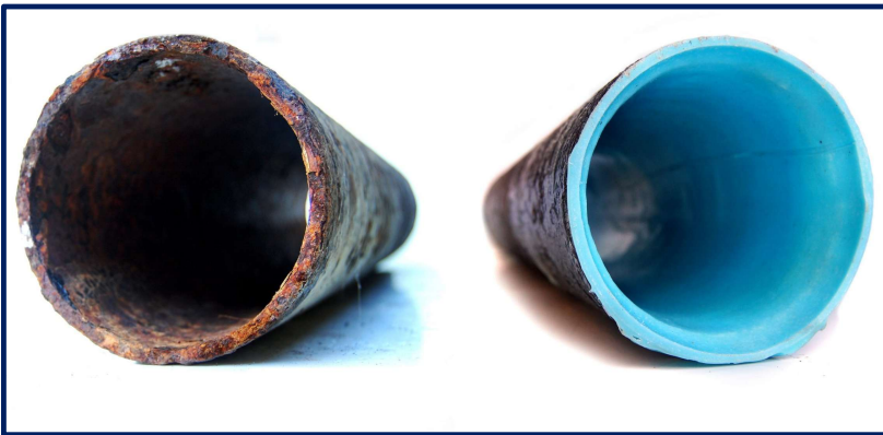
Example of pipe before and after CIPP via NuFlow Technologies
