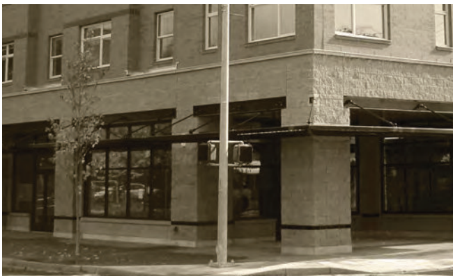
Public entries that are poorly defined or difficult to locate.
