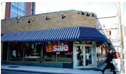
Horizontal window bands rely on hidden structural beams to span long openings. These arrangements lack visual support for the stories above.
