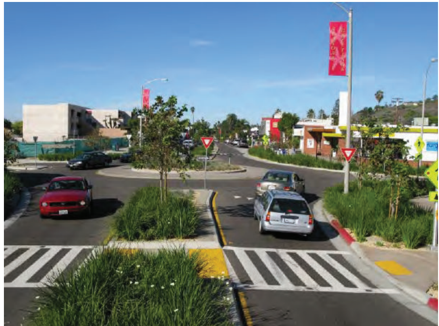
Roundabout: San Diego, CA (Credit: Michael Wallwork)
