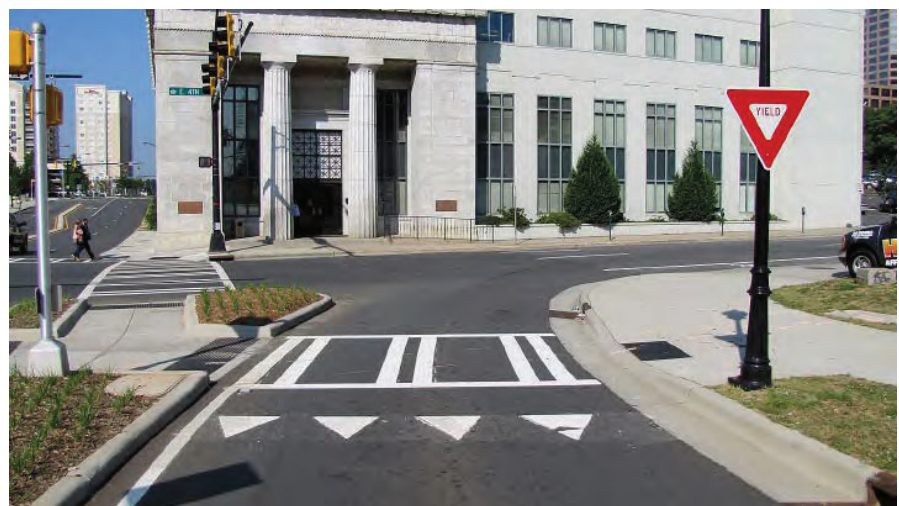
Multiple tools can be employed to improve uncontrolled crossings (Credit: Dan Burden)
