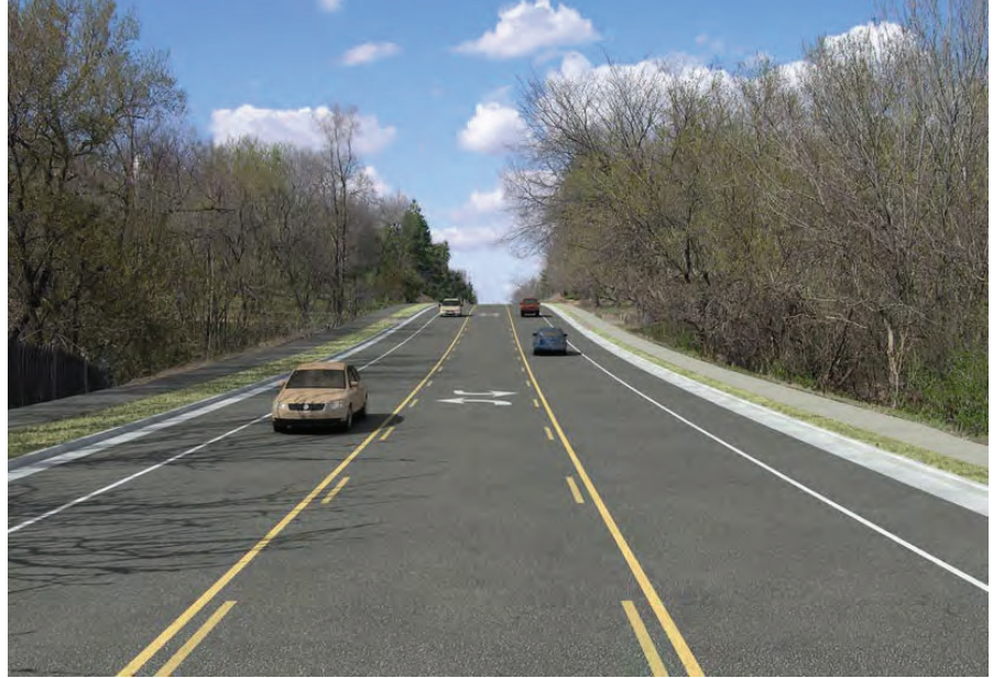
Center-turn lane (Credit: URS)
