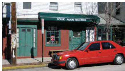
Blank walls and windows are uninteresting and shoppers may pass on by.
