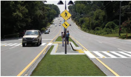
Staggered median crossing (Credit: Marcel Schmaedick)
